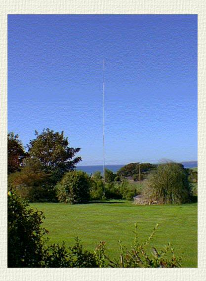
The HF2, is about 30ft long, and has an L/C band switching arrangement near the base. This L/C circuit consists of two coils in series, and a "doorknob" capacitor in parallel with the lower, larger coil. I'm reluctant to call this L/C arrangement a "trap", as it appears to operate in a different manner to the "traps" we see in antennae like the W3DZZ. If my analysis is correct, it appears to work in the following manner...
